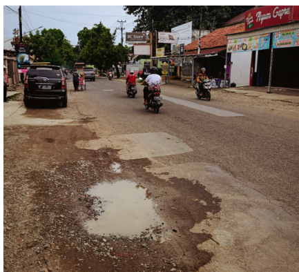
Figure 9. Potholes
